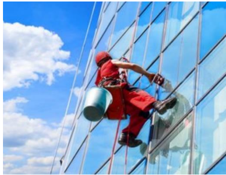
Figure 1. Worker working at height to clean windows
